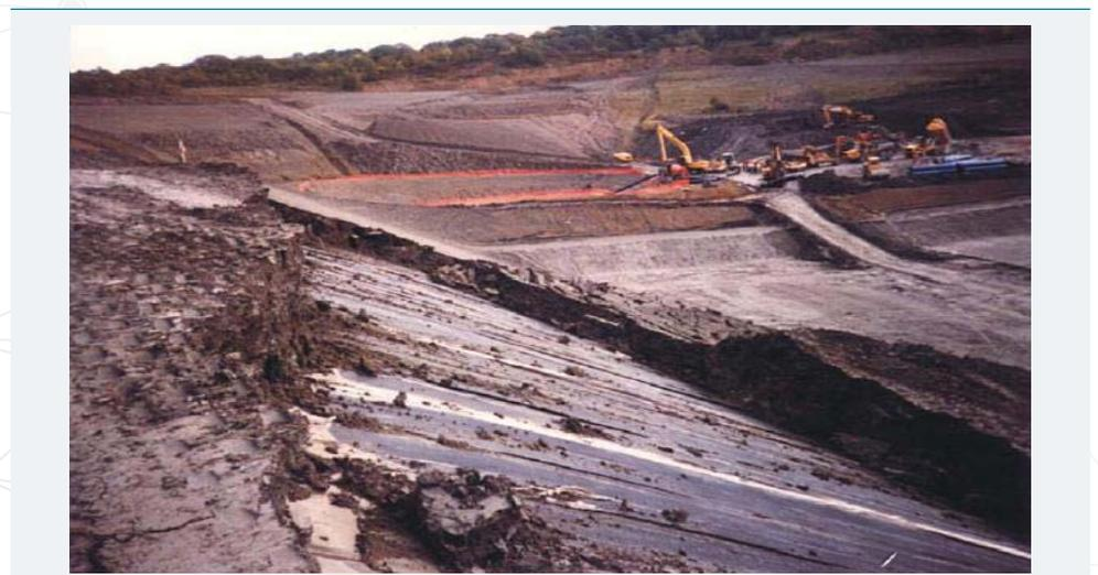
Figure 5: Shallow Translational Failure in Cover System [8].
